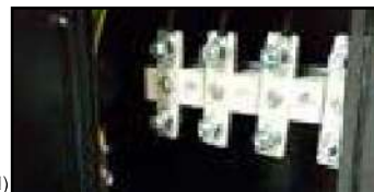
Earth Connection Plug (inner side Control Panel)
